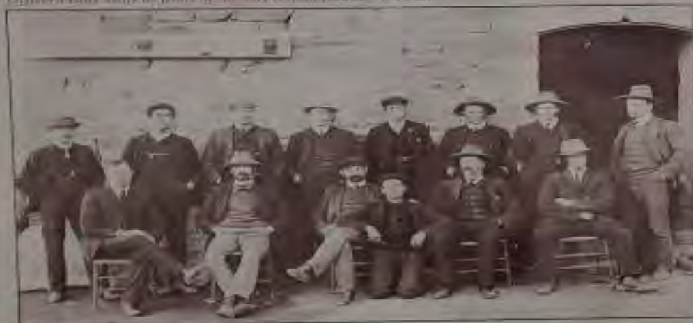
OFFICERS AND MEN OF THE CIVIL ENGINEERING CO. 1907
