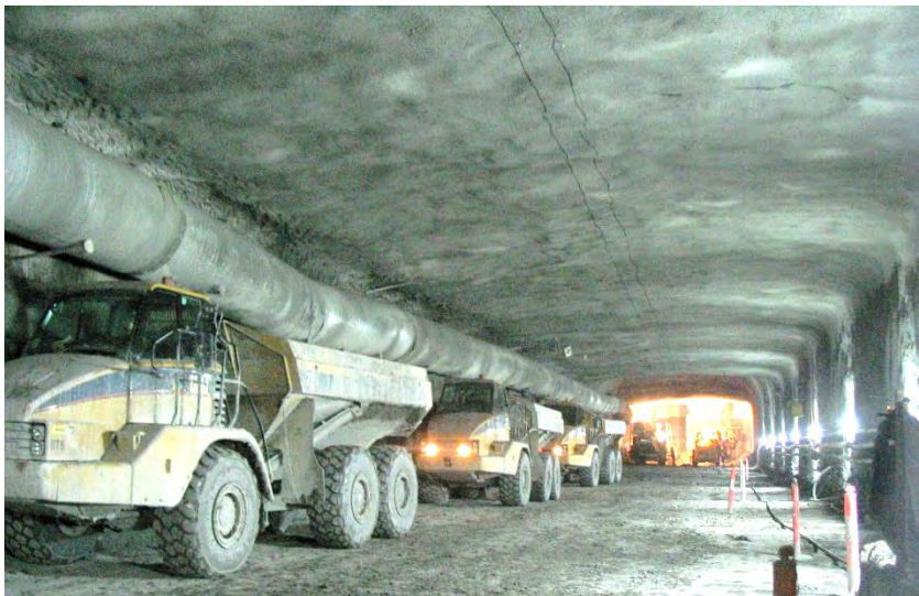
3-lane 12 m wide road tunnel. Lane Cove Tunnel, 2006
