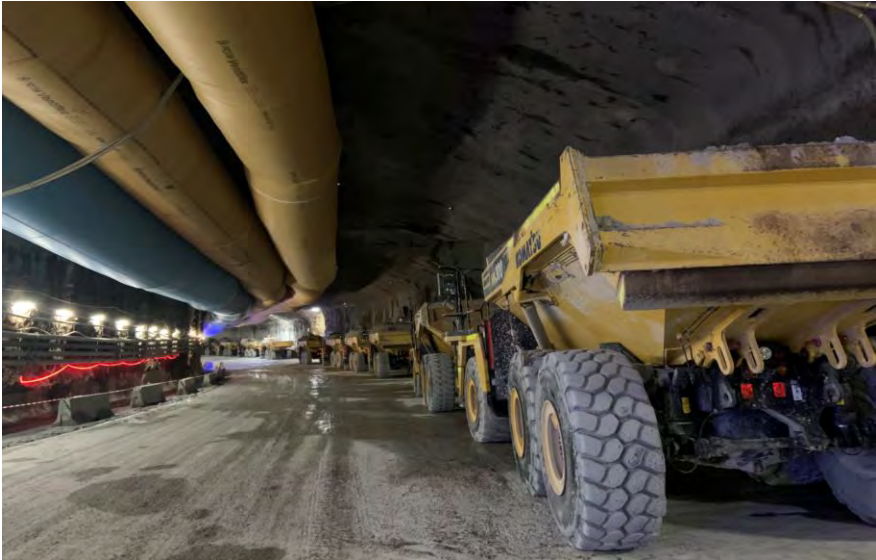
Convoy of trucks to service 18 roadheaders, RIC, 2022
