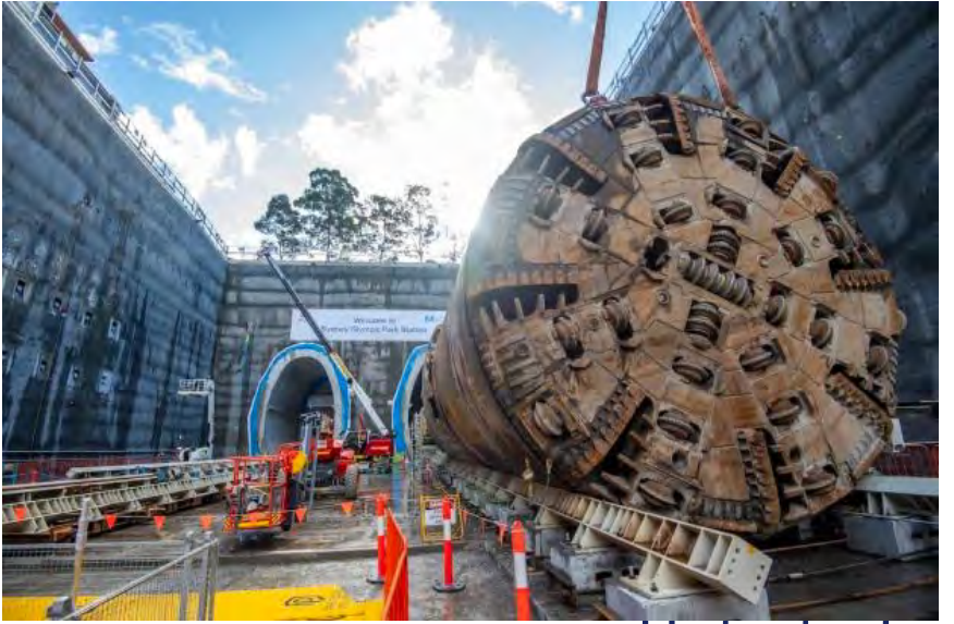
TBM, Sydney Metro West, 2024
