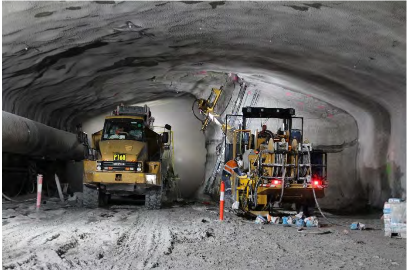
3-lane 15 m wide road tunnel. WestConnex 1B, Haberfield, 2018
