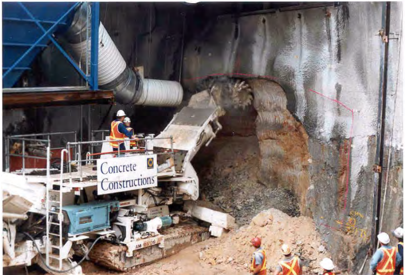
2-lane 8 m wide ramp tunnel. Eastern Distributor, 1998
