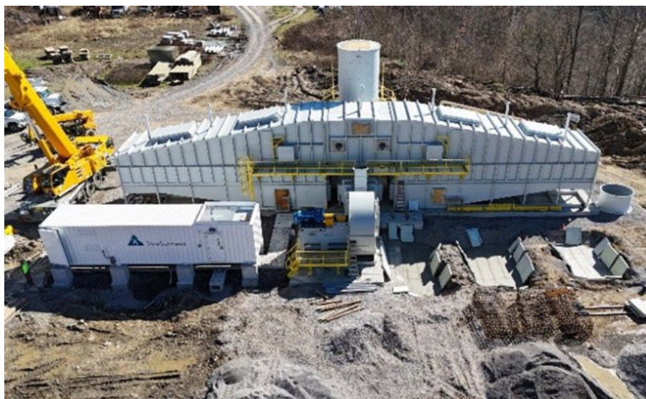
FIG 6 – Second VAMOX® unit of 258 000 m 3 /hr capacity (2022).
