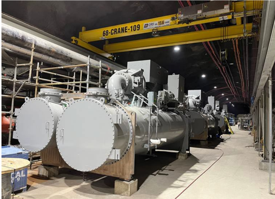
FIG 4 – Refrigeration plant room following completion of chiller installations.
