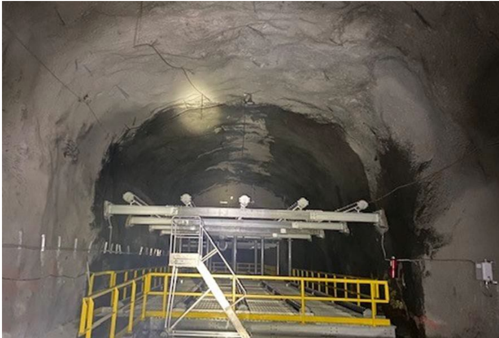
FIG 6 – View of CSC pipes, pipe supports and access platform following construction.
