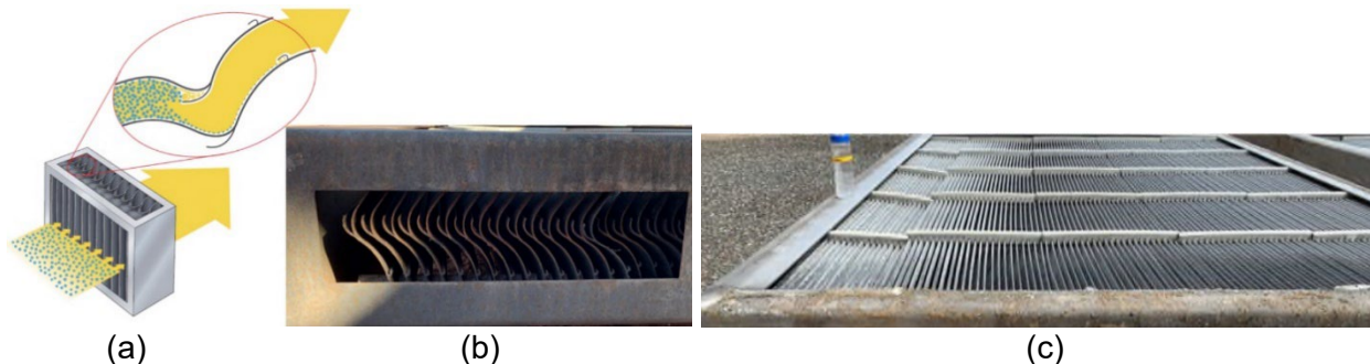
FIG 4 – Principle and photographic views of the mist eliminator panel: (a) Principle; (b) Mist eliminator side view; (c) Mist Eliminator isometric view.
