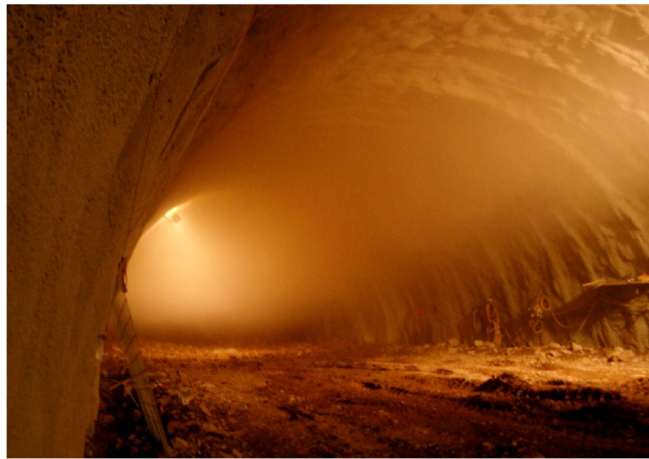
FIG 1 – Blast fumes in a roadway. Nitrogen oxides are visible as yellow/brown colour (image courtesy of Euromines).
