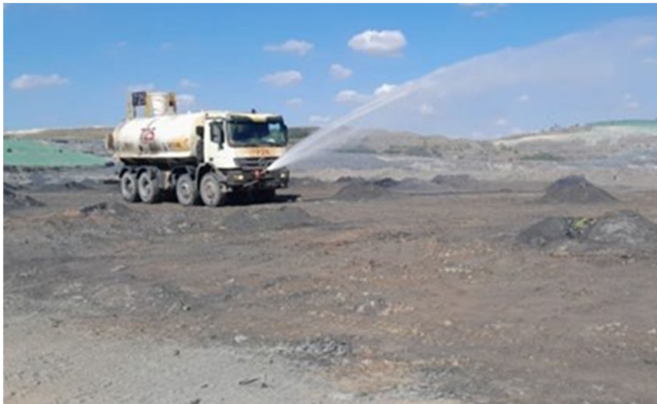
FIG 3 – Truck spraying water on the loaded blast pattern.
