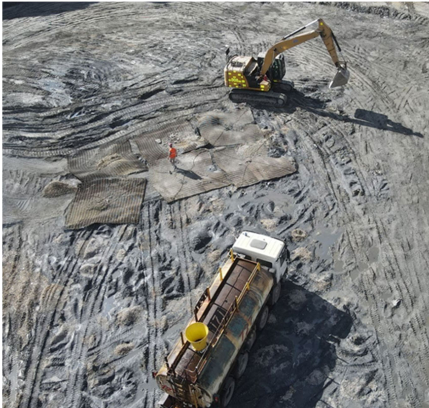
FIG 1 – Watering and placing mats on a WebGen™ blast.
