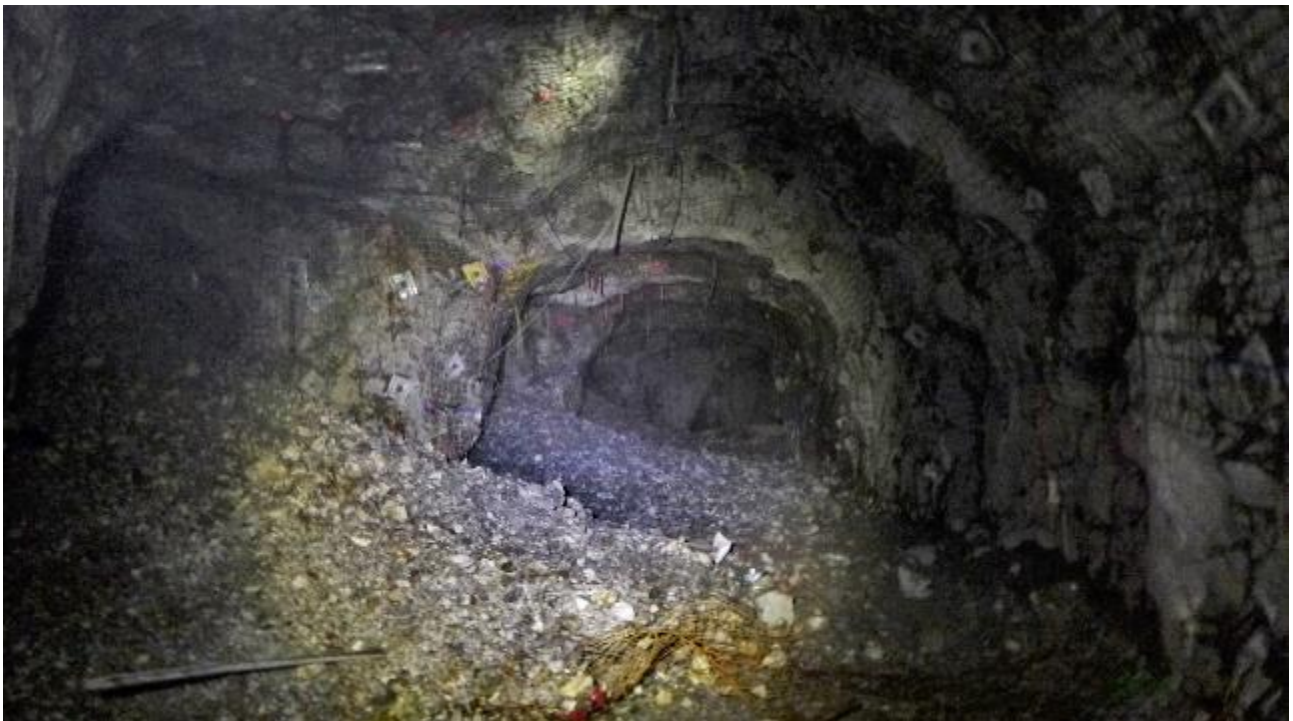
FIG 5 – JD 715 looting along the access past the three cross cuts after the 1 st firing
