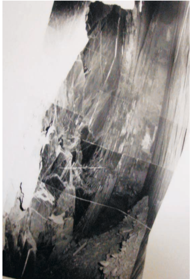
FIG 7 - A large structurally-controlled hangingwall failure.
