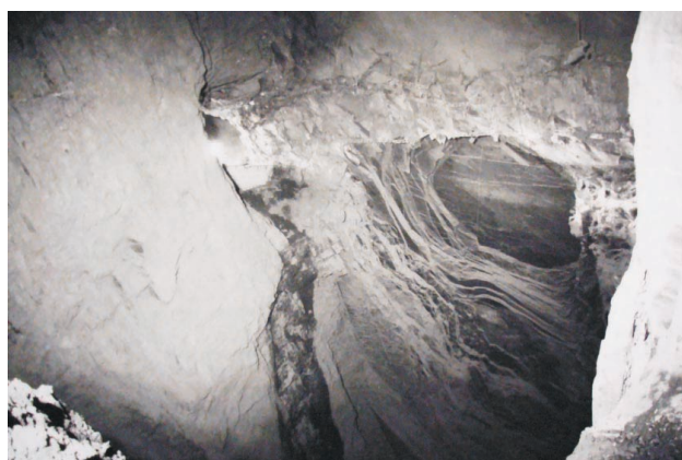
FIG 8 - A large stope hangingwall failure arrested by a row of cablebolts installed prior to stope firings.
